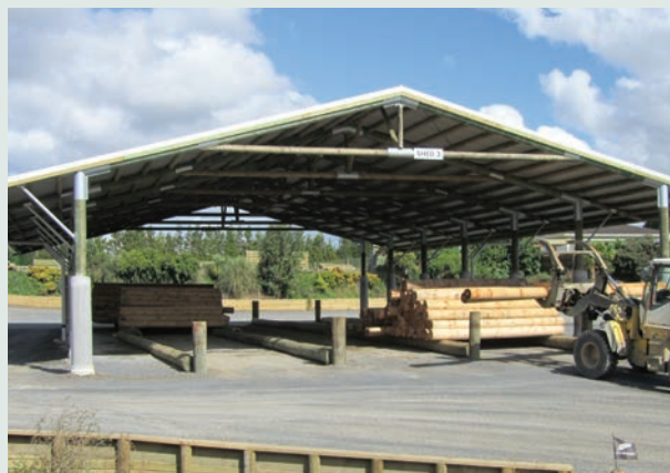
UniLogs used in an industrial shed.
